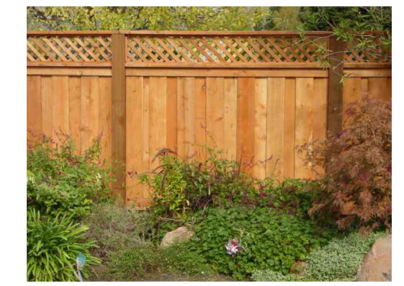
6' WOOD DOUBLE LATTICE TOP FENCE AT CORNER LOT SIDEYARDS & STREET FACING CUTOFF FENCES
