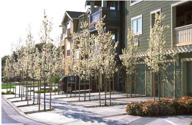
MULTI-FAMILY BUILDINGS FACING PRIVATE STREET
