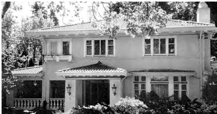
DISTINCT ENTRY EXTENSION
