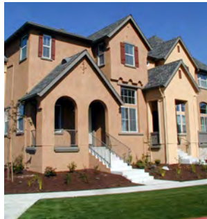
STEEPLY PITCHED ROOF
