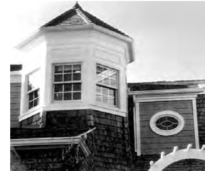
TOWER AND ARTICULATED WINDOWS
