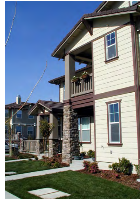
WOOD AND STONE COLUMNS
