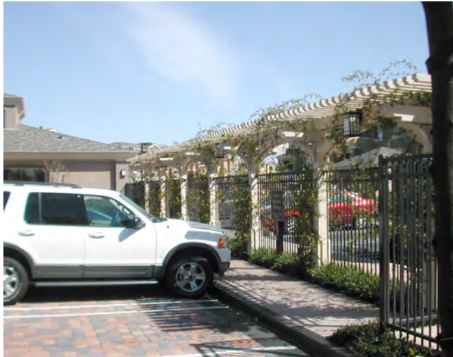
TRELLIS AT PARKING
