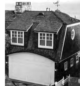
DOUBLE DORMERS ABOVE GARAGE
