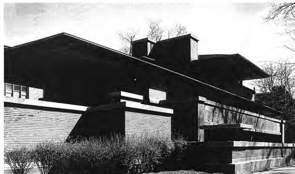
USE OF HORIZONTAL FORMS
