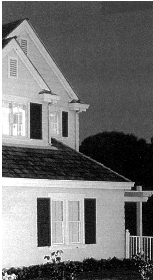
2ND FLOOR PUSHED BACK
