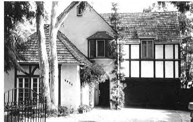
STEEP ROOF LINES
