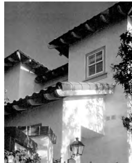
EXPOSED RAFTER TAILS
