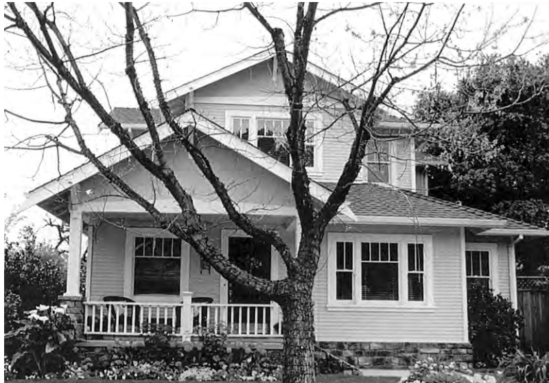
2ND FLOOR PUSHED BACK
