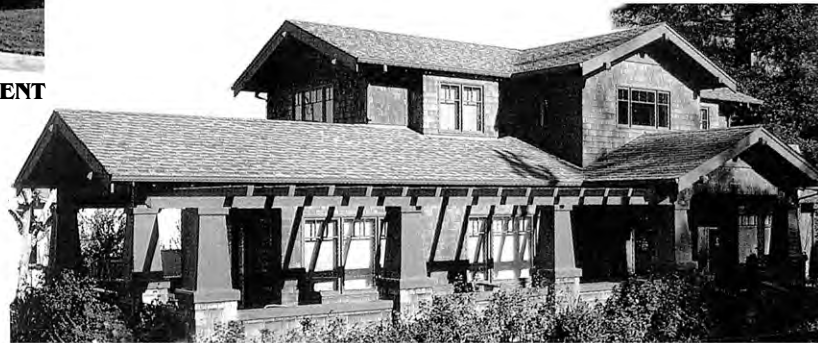
PORCHES WITH WOOD COLUMNS
