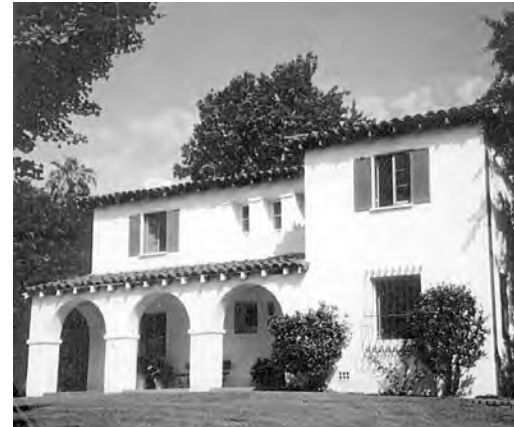
SHUTTERS AND GRILLES
