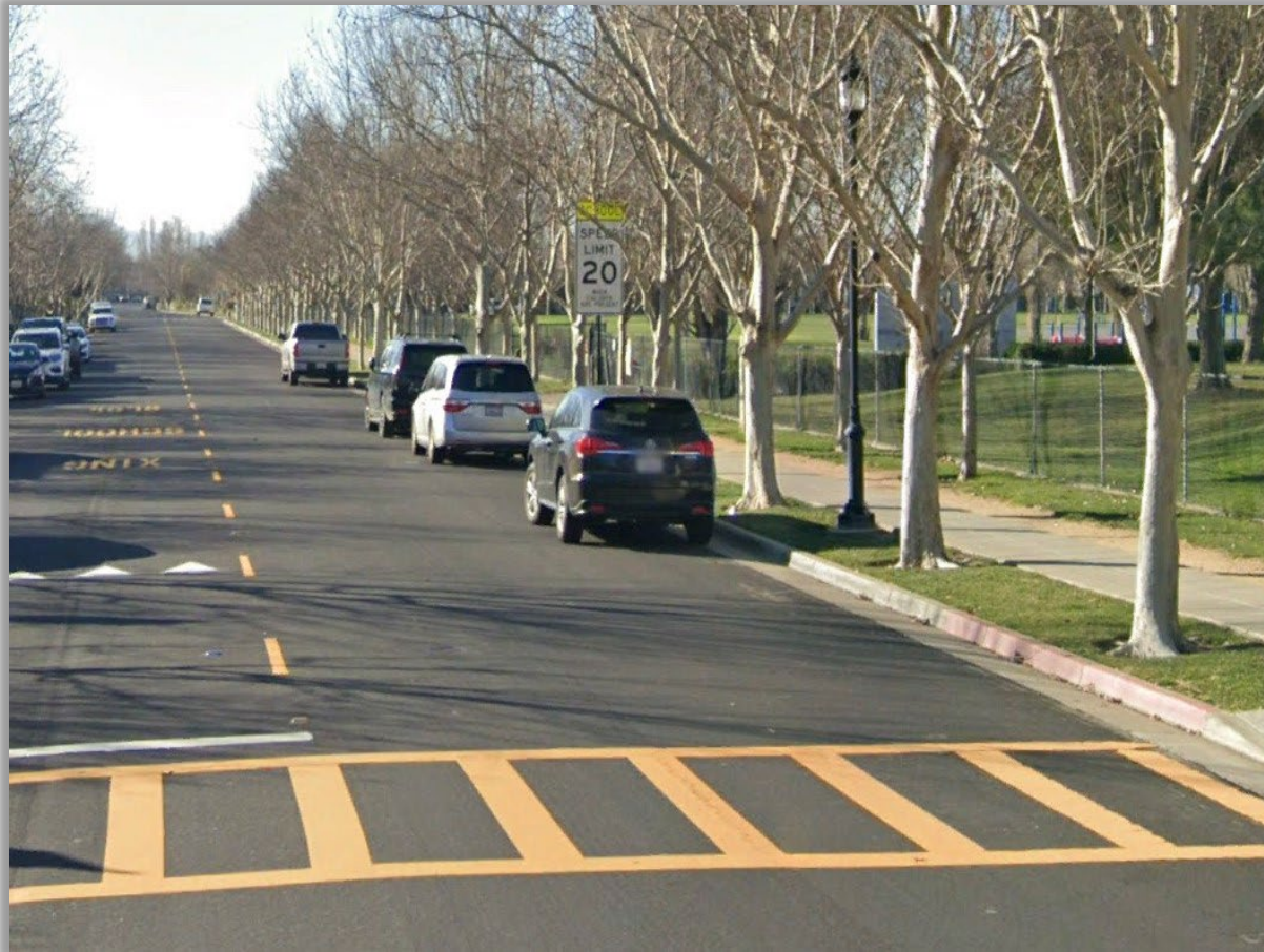
High Visibility Crosswalks and Speed Limit Signs
