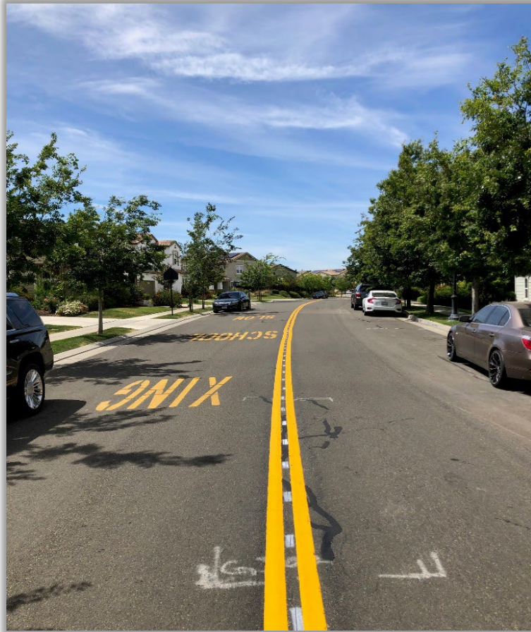
Tramonto Drive– Centerline Striping
